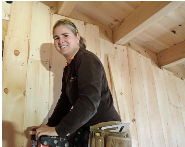
Staff carpenter Emma Woodward working on the paneling in the new Carriage Barn.
