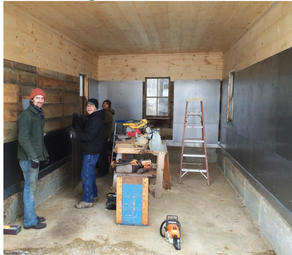
Jake, Ray & Brian putting up metal sheeting in Bernice's Garage.
