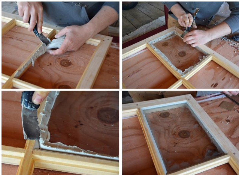
Steps in glazing from upper left: applying the initial layer of glaze putty is called bedding the glass; applying a top layer of glazing putty after setting the glass in place; cutting a clean bevel around the glass and removing excess putty (not shown is removing the excess putty from under the glass); and finally the glazed pane.
