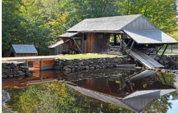
Fully repaired lower spillway.
