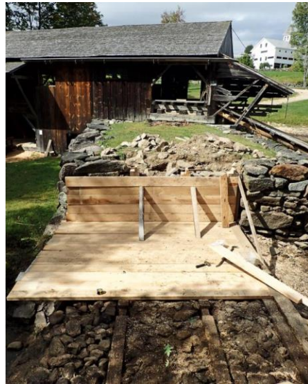
New floor and wall in process.
