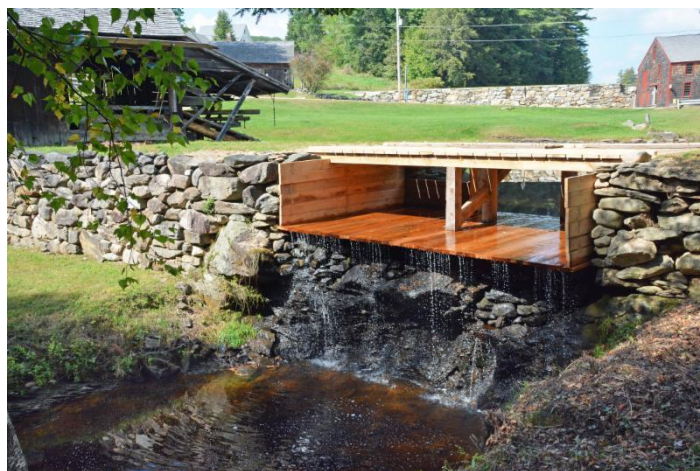
Completed spillway from the "toe end" downstream side.
