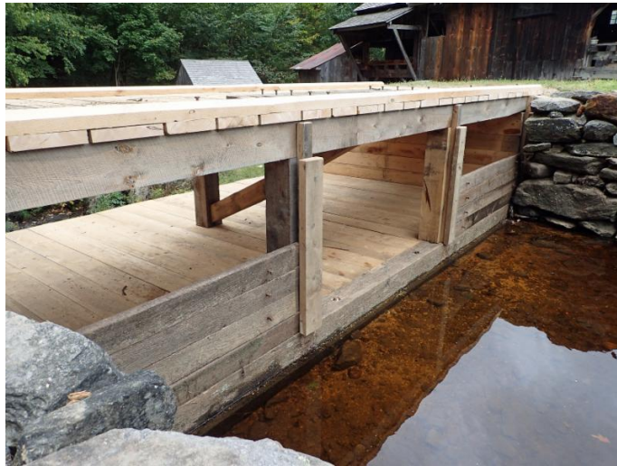
Completed spillway from the mill pond side.
