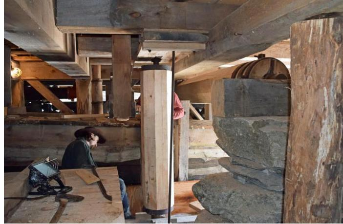
*Brian and Jake installing the shaft under the grist mill. (Photo BG)*
