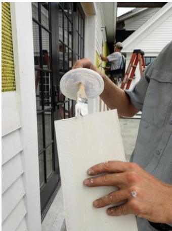
Painting the ends of a modern clapboard.
