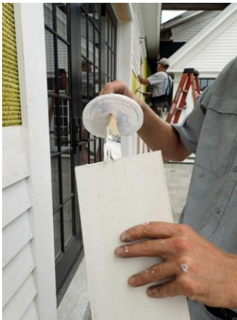
Painting the ends of a modern clapboard.
