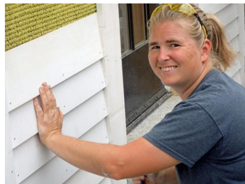
Carpenter Emma Woodward placing clapboards on the new Carriage Barn.
