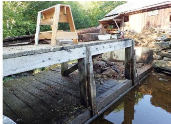
Stop logs (left) spillway deck and floor being removed for repair (right)
