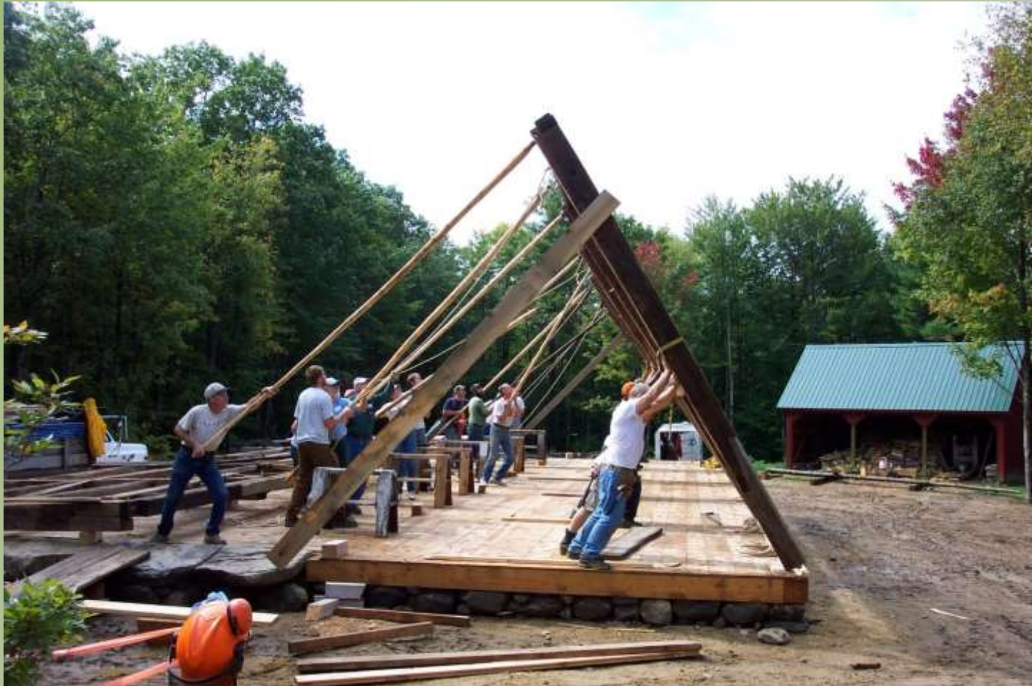
Raising the first side bent with gin poles
