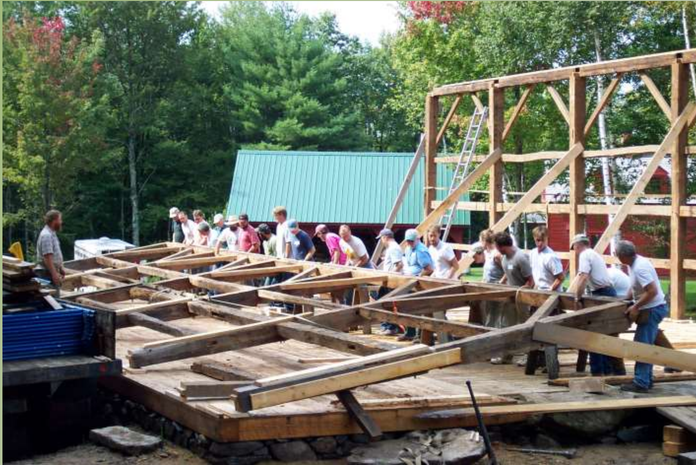
Raising the second side bent with gin poles
