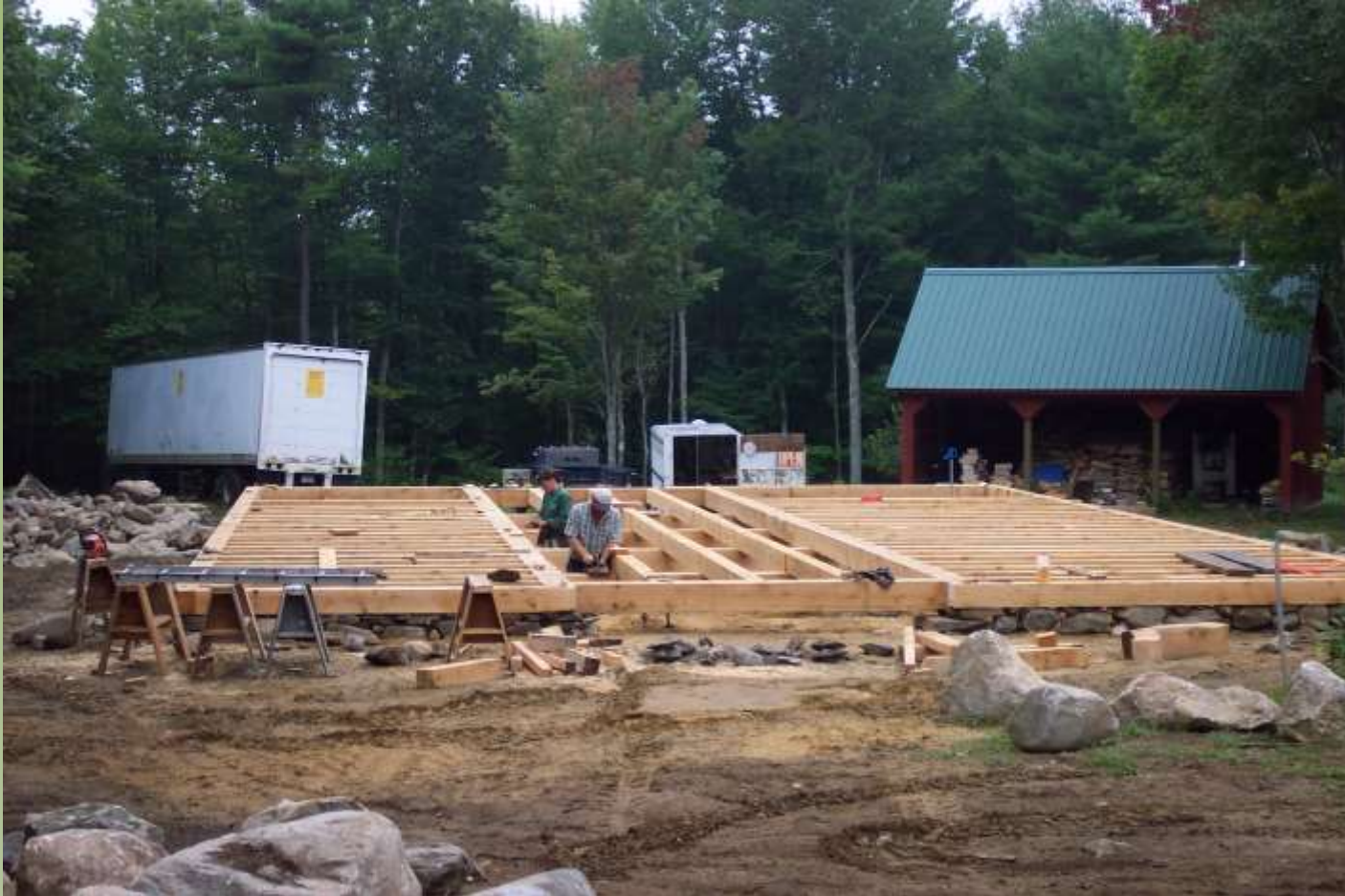
Laying out the timber framed floor system
